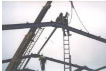
Roof being raised
