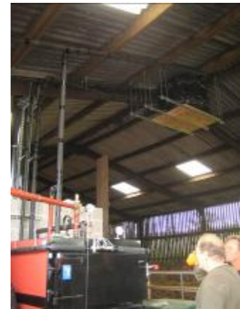
Installation of boiler above and cylinder below
