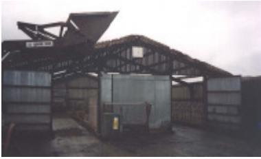
Cubicle shed before the roof was raised
